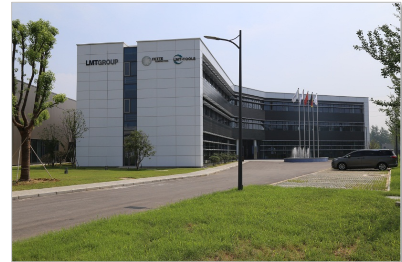
FCN – new Plant: Office Building
