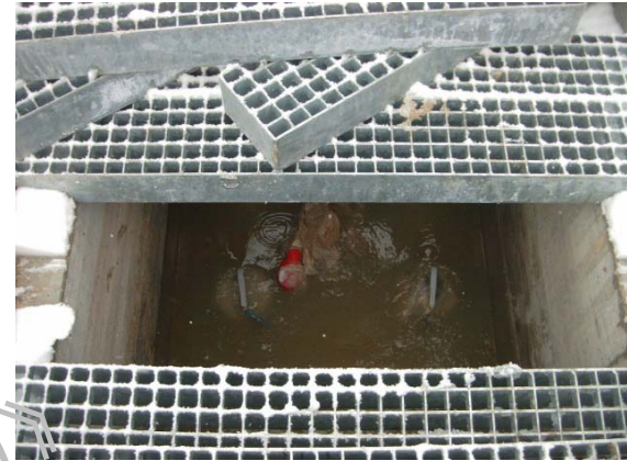
Waste water treatment plant / High density of big and dry particles at the Inlet of the Plant
