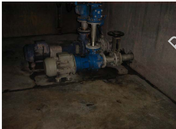
Waste water treatment plant / replacement of a Mono-Pump pumping sewage
