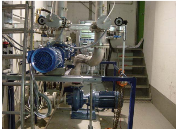
Waste water treatment plant / replacement of a Mono-Pump pumping sewage
